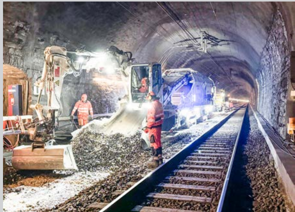
↳ Projekt Lötschberg Summit Tunnel Location: Bernese Oberland – Valais, Switzerland Client: BLS AG Scope: Conversion of 1.5 km of double track with four turnouts from ballasted track to slab track Construction phase: April to June 2024
