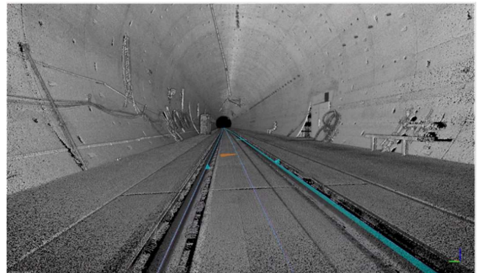
The output from a laser scan of a rail tunnel.
