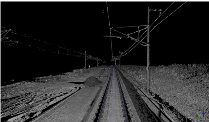
The output from a laser scan of a rail line.
